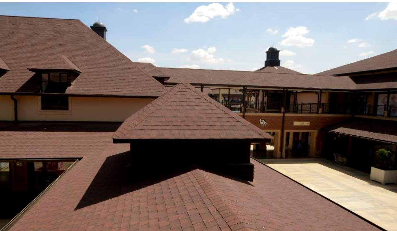
Roofing Shingles (Cambridge Xpress) Project - The Hub-Karen, Nairobi
