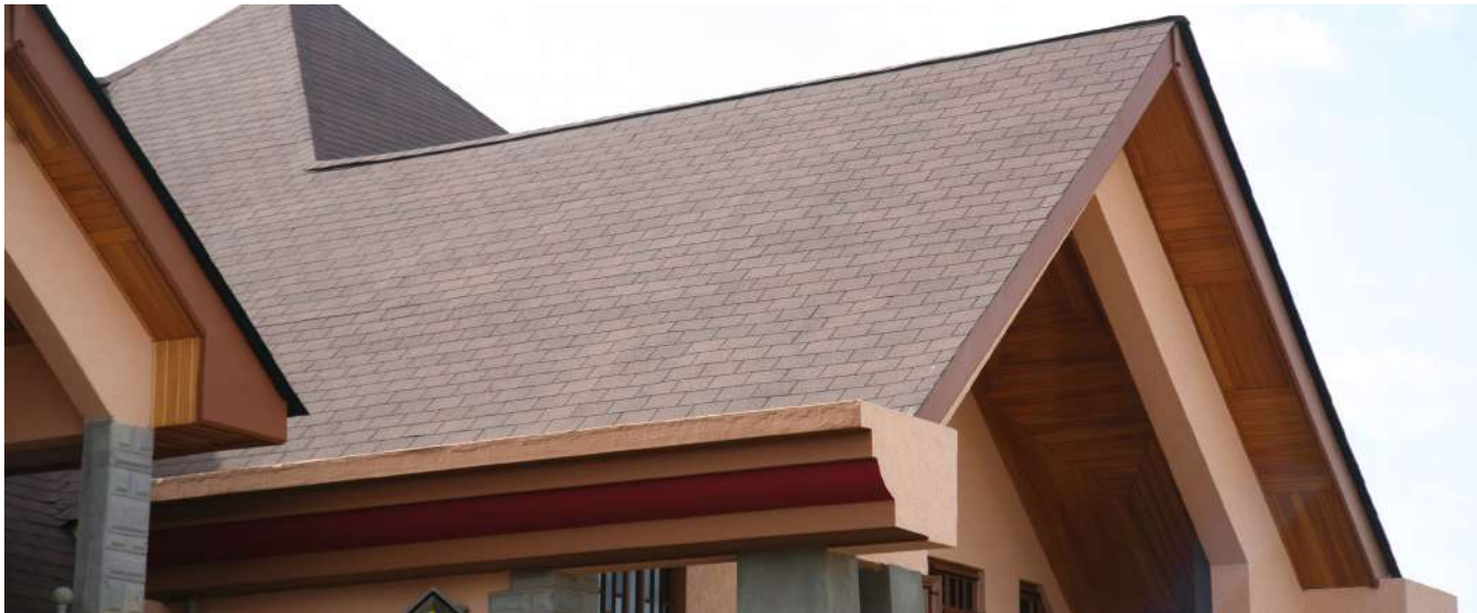
Roofing Shingles Project - Runda
